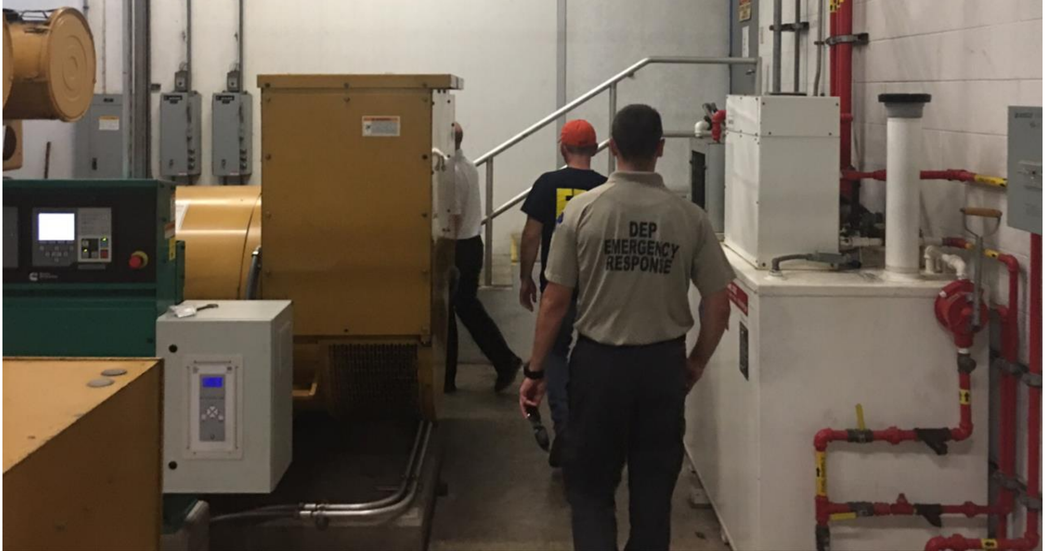
FDEP and EPA assessing Collier County Drinking Water Plant
