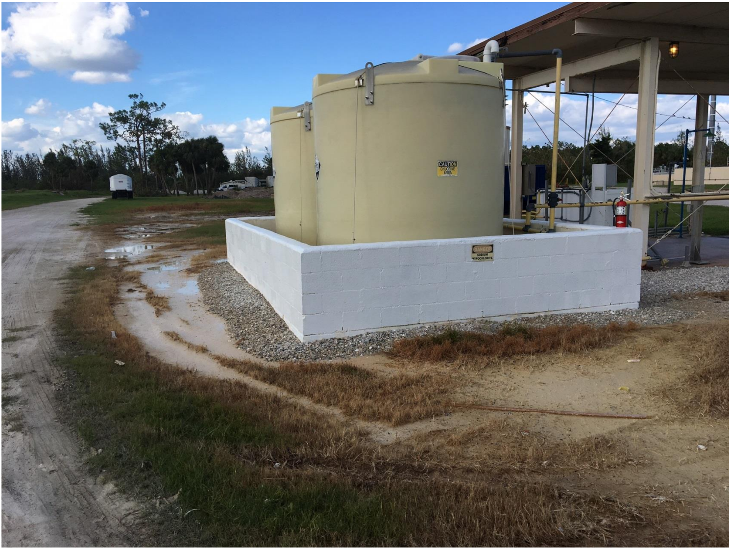
Sodium hypochlorite spill at WWTP
